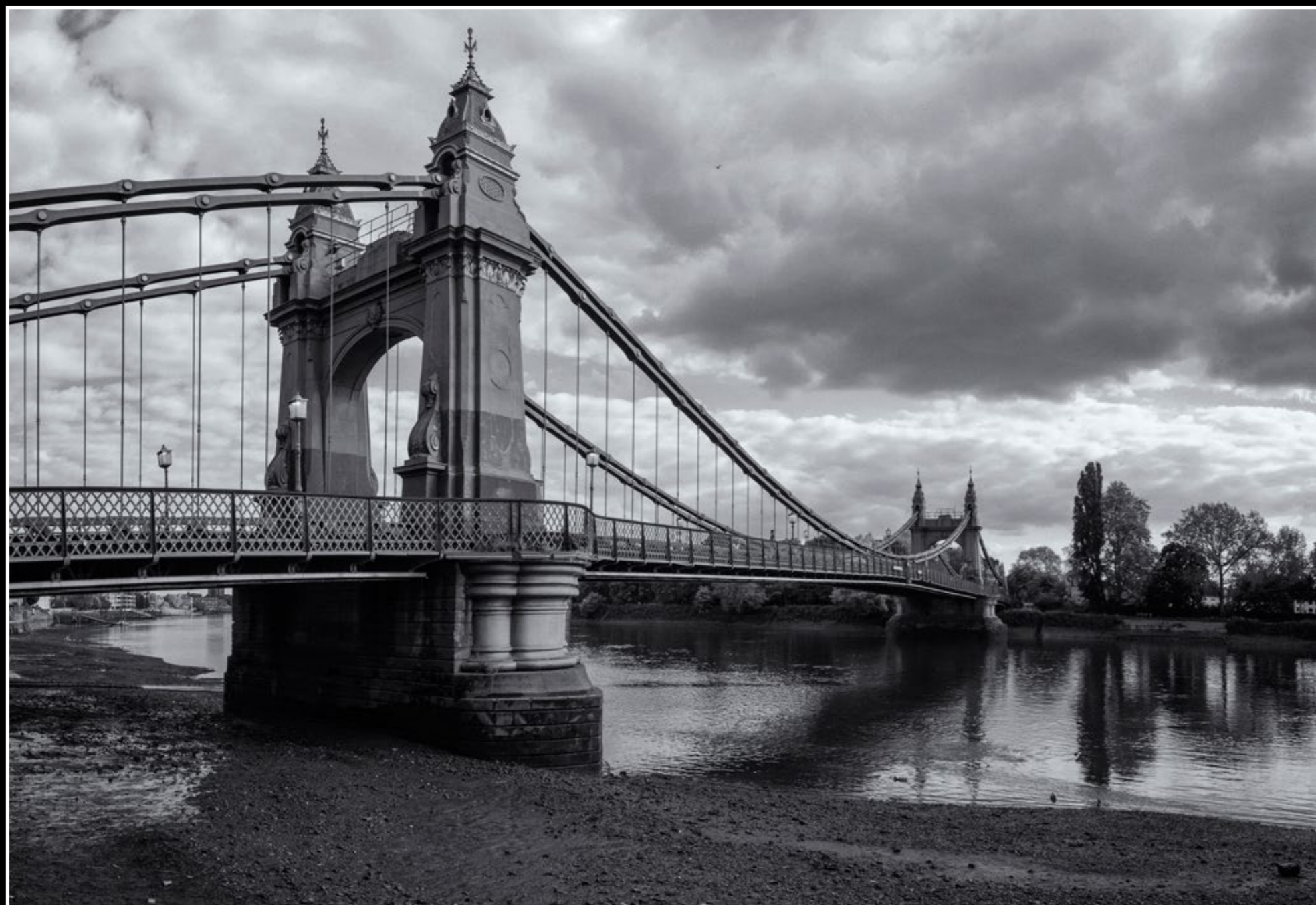
Hammersmith Suspension Bridge • London
